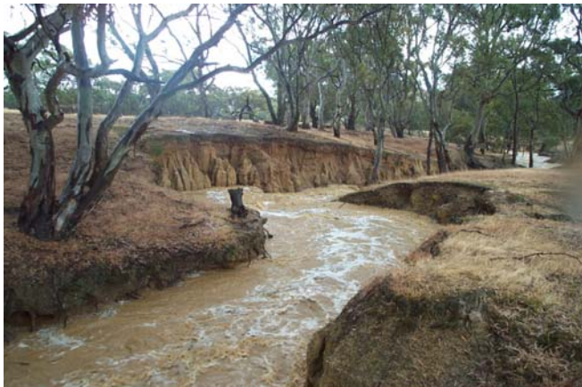
Erosion, transport and deposition of sediment in an erosion gully, Ararat, 2004. Photographer: Clem Sturmfels, DPI.
