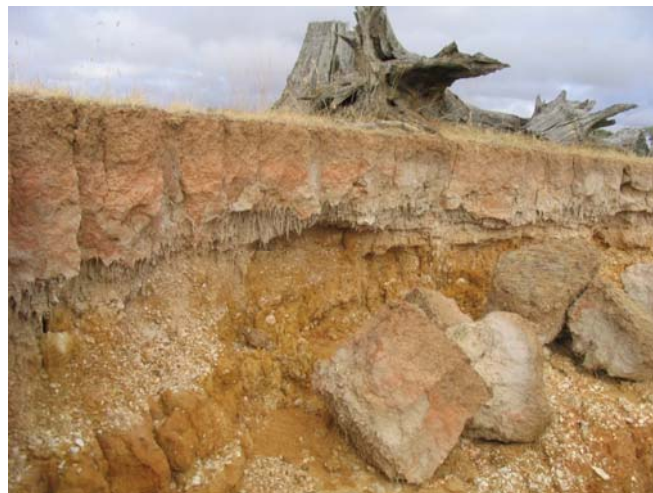
Bank erosion caused by slaking and blockfall, 2004. Photographer: Clem Sturmfels, DPI.
