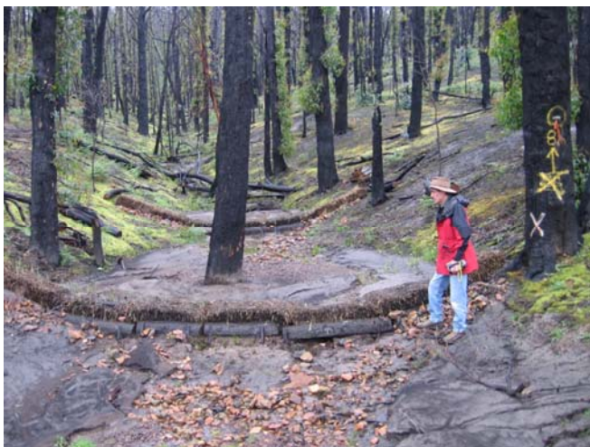
Above: A successful straw bale and log sediment trap in a steep site, St Andrews, 2009. Photographer: Tim O'Donnell, Nillumbik Shire Council.
