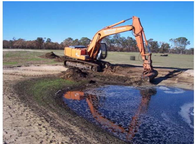
Removing fire sediment from farm dam, Grampians, 2006. Photographer: Clem Sturmfels, DPI.
